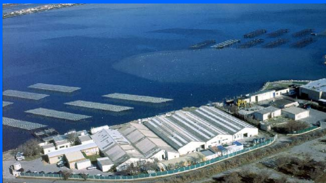
Aquaculture research facility
